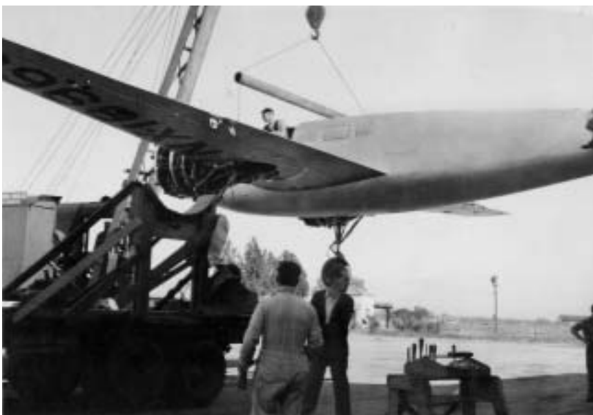
The BTC-1 on the sling, about to be positioned sideways on the truck.
