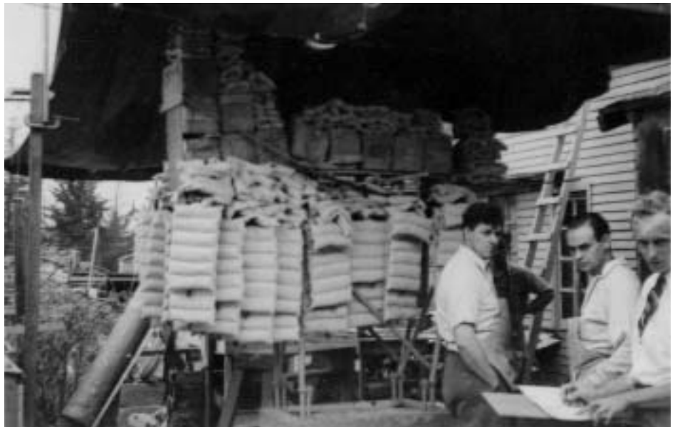
Proof loading of the wing structure being done with the then state of the art. Sand bags were piled on top of the structure until it failed. Hawley Bowlus is seen on the left. Other people in the photograph are not identified.
